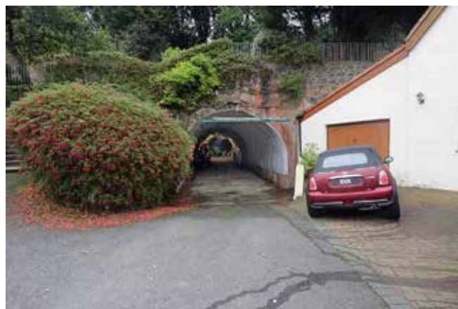
The north entrance to Ho 3 on Havelet
